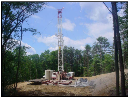
CSi's Rig #2 Drilling Reserve's Olian #3 in Kanawha County, WV in 2005
