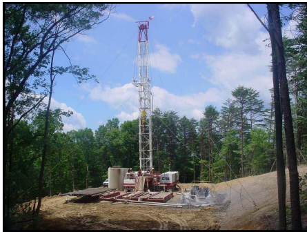
CSi Rig #2 Drilling Reserve's Olian #3 in Kanawha County, WV in 2005
